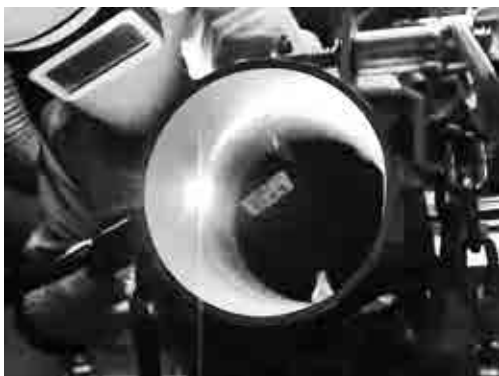
Figure 1: Site welding by TG-X filler rod
