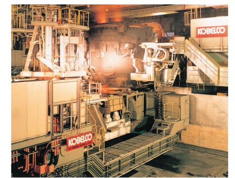
Continuous Casting Equipment
