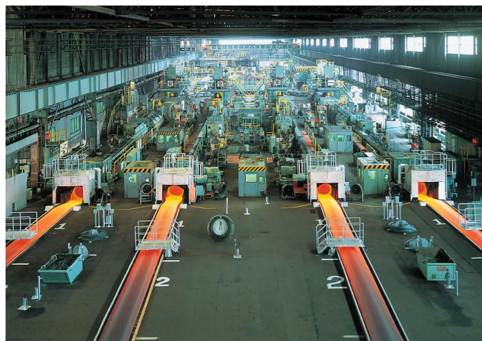
No.8 Wire Rod Mill
