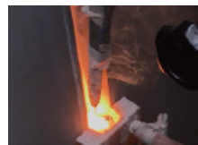
立向自動溶接 Vertical Up Welding
