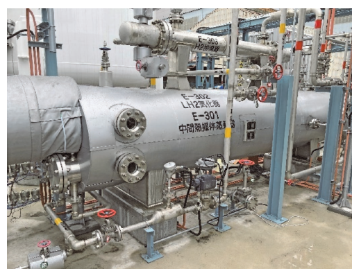
図2 実証用IFVの外観 Fig.2 Outside view of IFV for LH 2 vaporization demonstration
