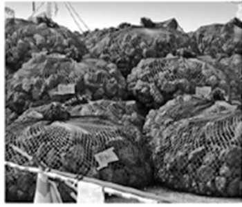
(a) Submerged breakwater construction materials (Steelmaking slag stone)
