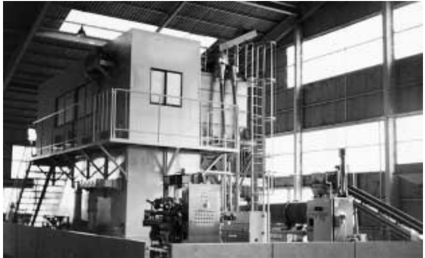
写真1 UBC 塗料剥離装置の外観 Photo.1 De-coating equipment
