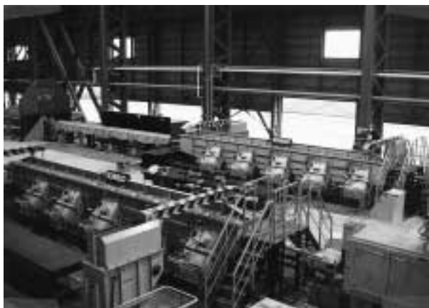
写真 3 仕上列 (S-HUM) Photo.3 Finishing mill (S-HUM)
