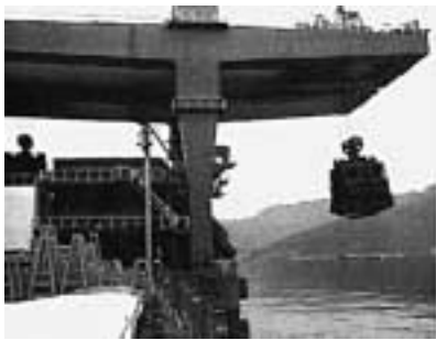
(Running Trolley with Winding Ropes)
