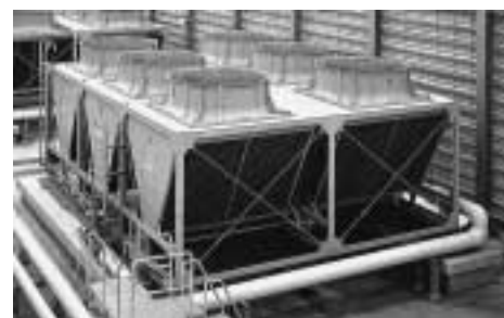
写真3 空気熱交換器外観図 Photo 3 Outside view of air heat exchanger unit
