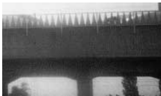
写真3 新幹線用山形防音壁 Photo 3 Mountain shaped barrier alongside Shinkansen Line
