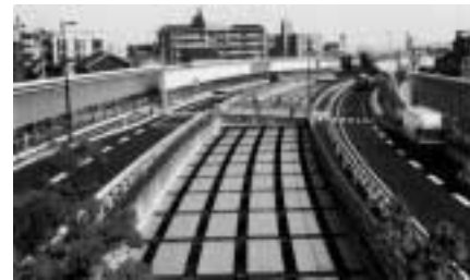
写真7 掘割り道路用水平吸音板施工例 Photo 7 Horizontal type sound absorbing panel units constructed over the trench type road
