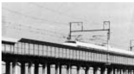
写真2 新幹線用張出し型防音壁 Photo 2 Overhanging type sound barrier for super express railway
