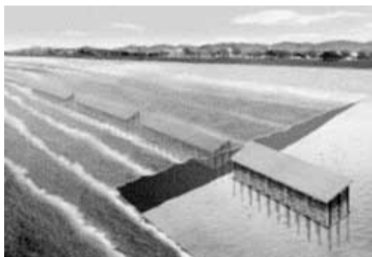
図3 空隙率傾斜型人工リーフ Fig. 3 Artificial reef with varied opening rate
