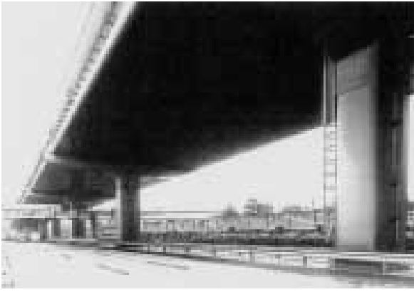
写真12 裏面吸音板 Photo 12 Sound absorbing panel under viaduct
