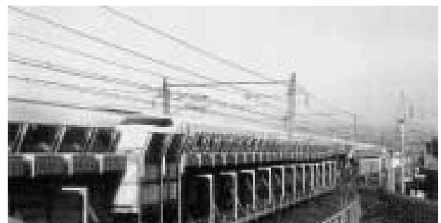
写真8 張出し型防音壁 Photo 8 Double sound barrier with extended plate and directivity plate
