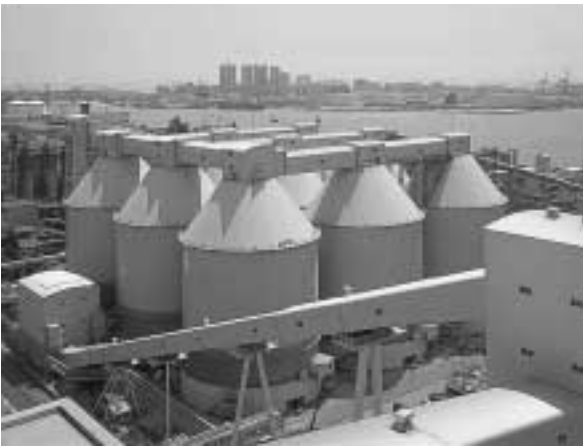
写真2 運炭貯炭設備 Photo 2 Coal silos and belt conveyor
