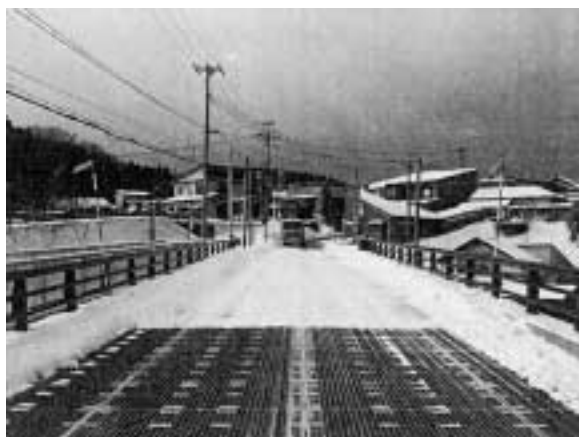
写真2 降雪時の路面状況 Photo 2 Bridge deck surface after snowfall
