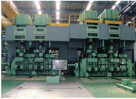
Roughing mill train
