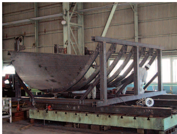
図11 鋼殻製作 Fig.11 Manufacturing of steel shell
