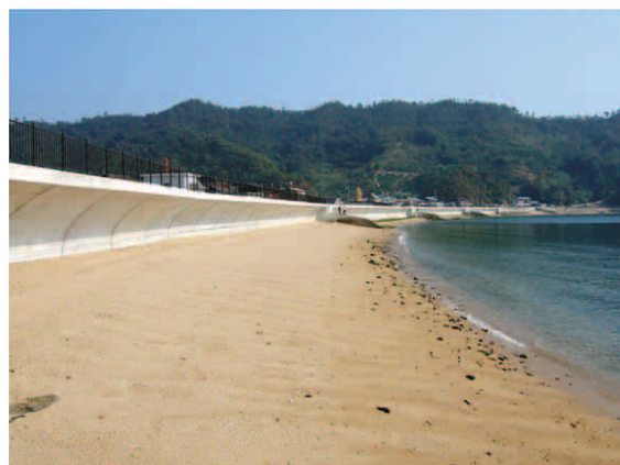
図14 完成 Fig.14 Completion
