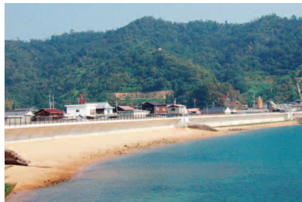
図1 フレア護岸の設置状況 Fig. 1 Installation of flare-shaped seawall
