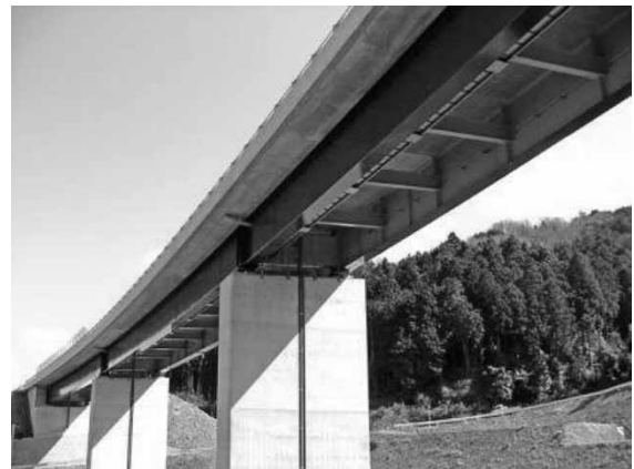
図2 南阪奈道路竹内橋 Fig. 2 Takeuchi-bashi Bridge of Minami Hanna Road
