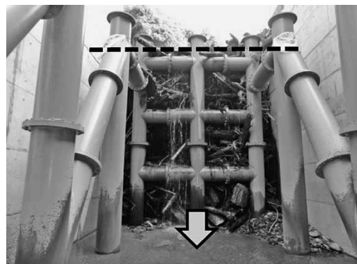
図10 土石流後の西谷川堰堤 Fig. 10 Nishitanigawa sabo dam after debris flow
