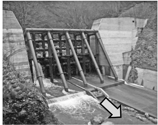
図13 二期施工後の野中沢第2堰堤 Fig.13 Nonakasawa 2 nd sabo dam after second phase
