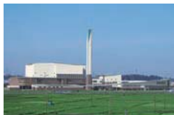
Heat recovery facility at the Shigenka Center, Kawagoe City
