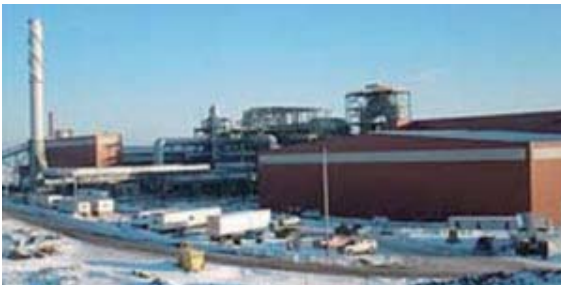
View of the world's first commercial ITmk3® Plant
