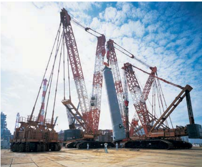
Ultra-large crawler cranes
