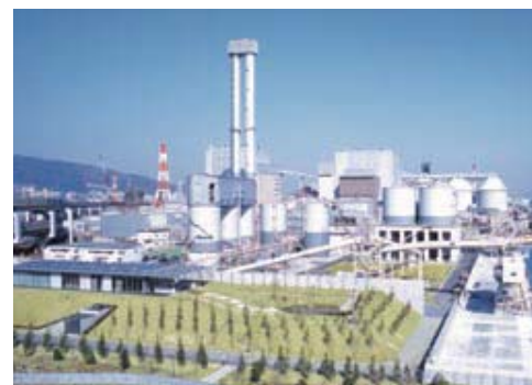
Shinko Kobe Power Inc.
