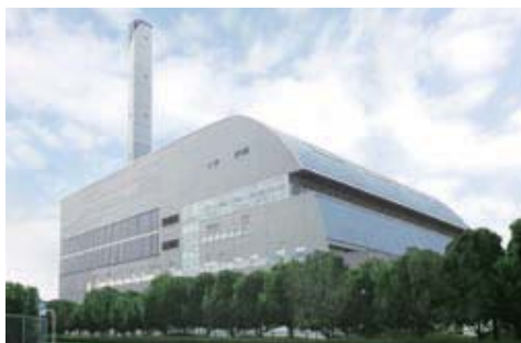
Minami Refuse Incineration Plant, Sagamihara City
