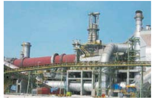
GIIC's No. 2 Pellet Plant
