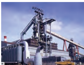
No. 3 Blast Furnace at Kakogawa Works
