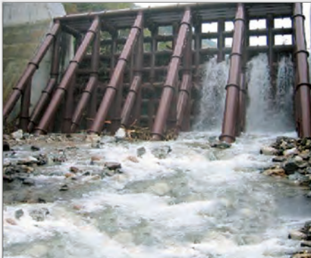
Steel Structures and Sabo Dams
