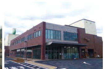
Haga Regional Waste Treatment Plant
