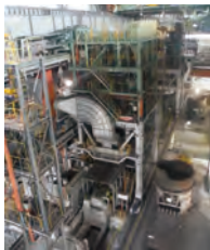
The new hot-metal treatment plant
