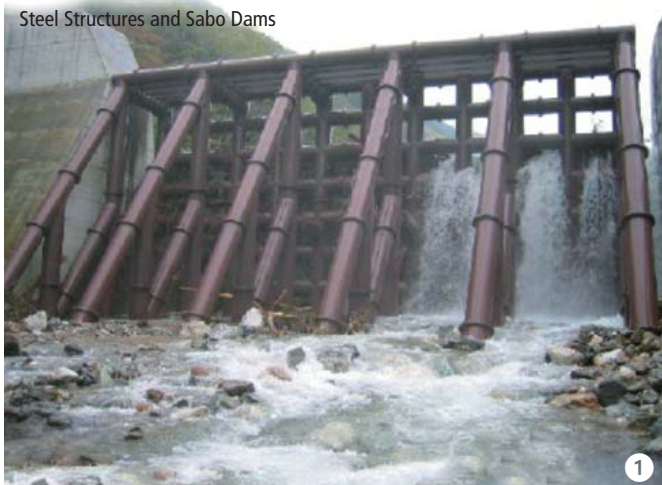
Steel Structures and Sabo Dams
