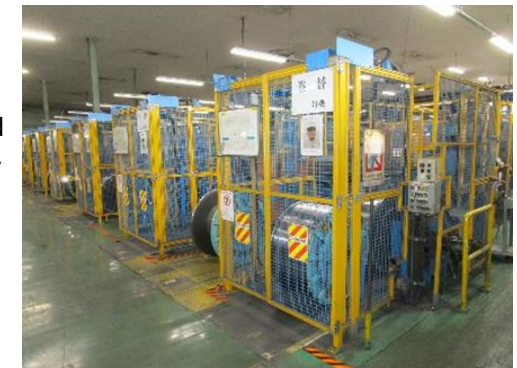
Welding division machine safety at Ibaraki Plant (Promote installation of safety fences, etc. with an interlocking function on moving parts)
