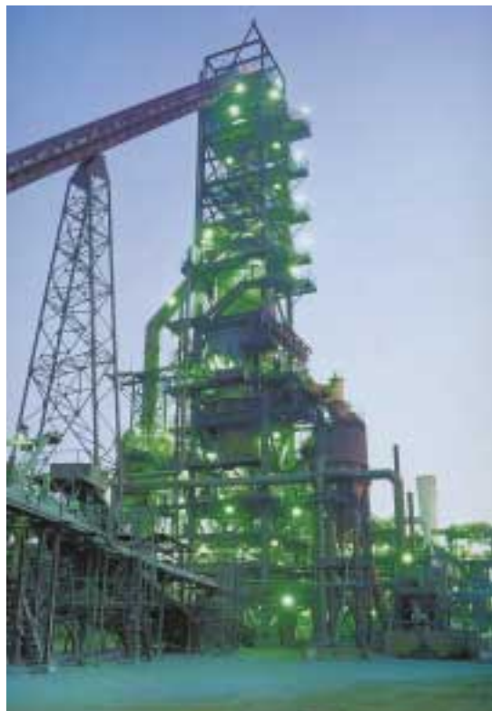
Direct-reduction iron-making plant
