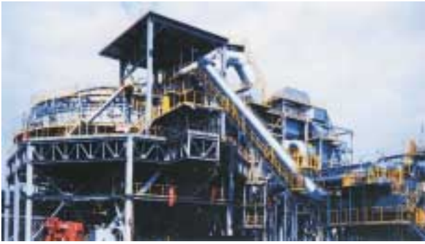
Photo 3 FASTMET commercial plant
