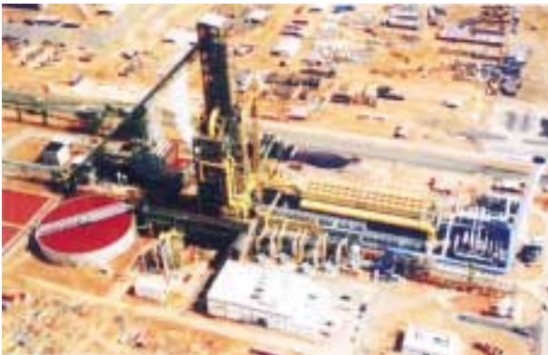
Photo 1 MIDREX DR plant
