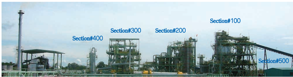
Fig. 4 Full view of UBC 600 tonnes/day plant
