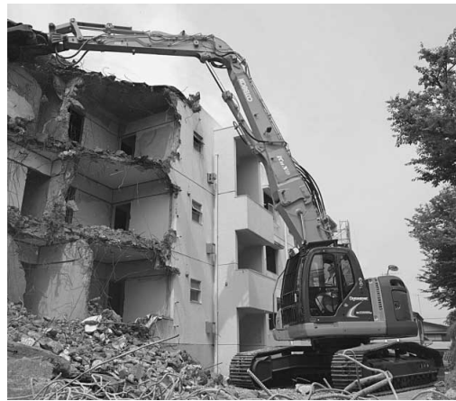
Fig.16 SK235SRDLC 2 piece ultra long attachment machine
