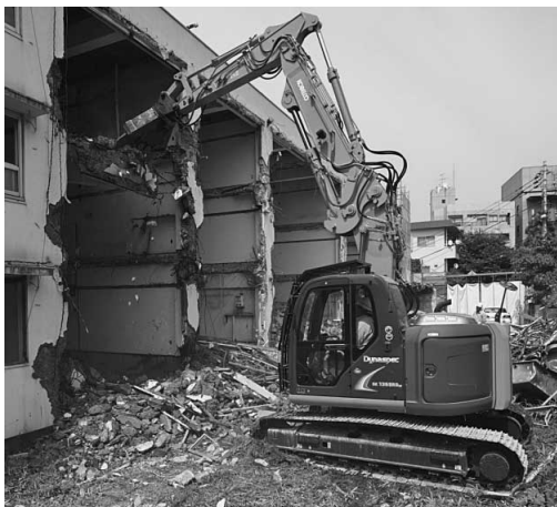
Fig.15 SK135SRDLC separate boom attachment machine
