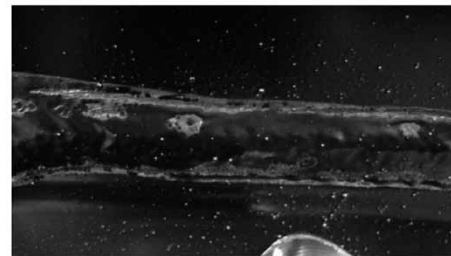
Fig. 6 Rust generated on the welded part after paint treatment
