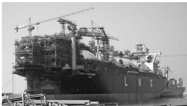
Fig. 6 Outside view of OLT FSRU (under construction)
