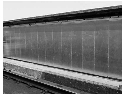
Fig. 9 Installation of microperforated aluminum sound absorbing panels
