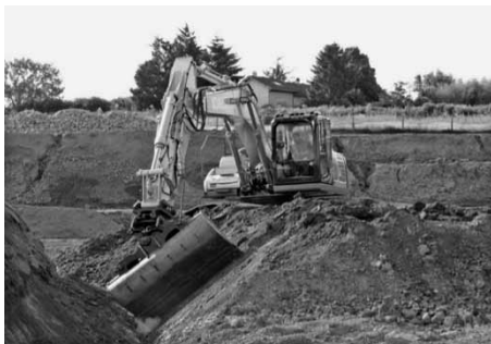
Fig. 9 Overview of SK200H-10 equipped with tilt bucket
