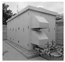
Fig. 3 Water-electrolysis hydrogen generator
