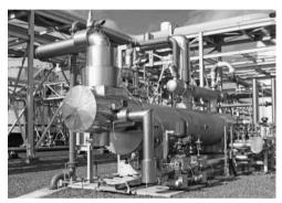
Fig. 8 Appearance of IFV for supplying cold energy to air conditioning apparatus in Kagoshima Terminal of NIPPON GAS Co., Ltd.
