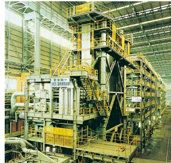
Continuous annealing facility
