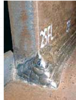
● Example of horizontal process (bead external view)
