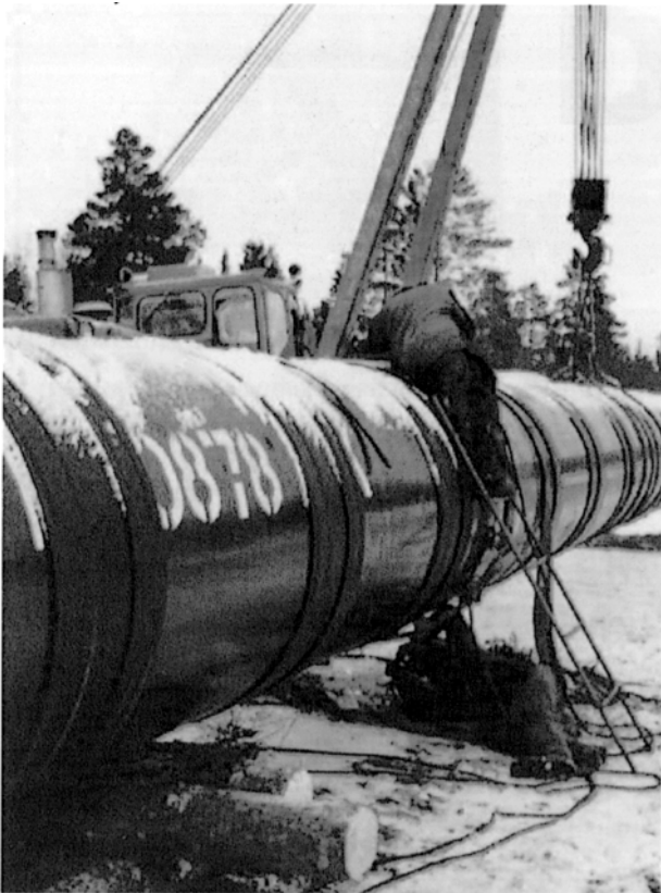
Fig. 3 — A pipeline-welding site in Russia where LB-52U is used for joining the girth joints in freezing weather
