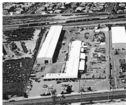
PIPE FAB in Santa Fe Springs, California (Left)
