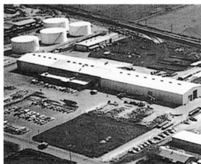
PIPE FAB in Salt Lake City, Utah (Right)
