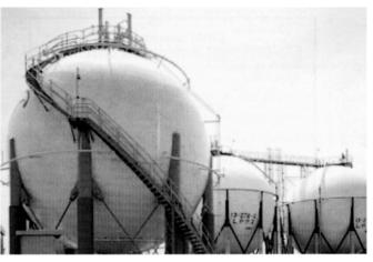
Fig. 1 — Some types of LPG storage tanks use ASTM A537 CI-2 steel having a minimum tensile strength of  $550N/mm^2$ , and LB-62L is one of the most suitable covered electrodes for this steel.
