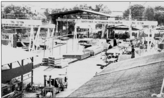
A TKI fabrication shop at the Batam Plant located on Batam Island in Indonesia
