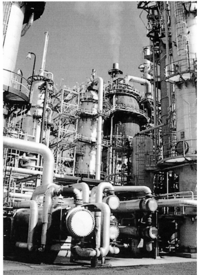
Photo 1. 1.25Cr-0.5Mo steel is used for applications operated at the temperatures from 350-550°C. For such high-temperature applications, the materials must metallurgically be stable, resisting elevated temperature oxidation and creep rupture. Kobe Steel has used its accumulated technical expertise to pursue quality control of TGS-1CM, maintaining its high performance for the piping of oil refineries and power boilers.
