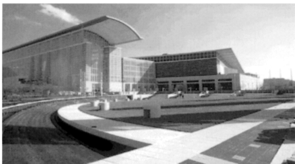
McCormick Place, America's premier convention facility, was the venue for FABTECH 2001 (Source: www.Mccormickplace.com )
