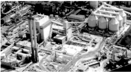
Fig. 1. 2.25Cr-1Mo steel is a must in a coal-fired power plant (A Kobe Steel's power plant under construction)
