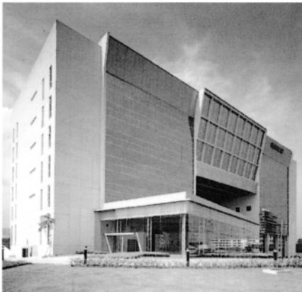
IMCT's head office rising high with much sunlight passing through its glass-rich structure in Phrapradaeng City, Thailand
