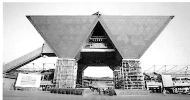
Japan International Welding Show 2002 was held at Tokyo Big Sight — the all-round convention facility having a huge floor area of 230,000 square meters (Courtesy of www.bigsight.or.jp)
