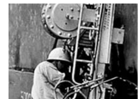
P3-7 Welding of crude oil storage tanks, Part 2
