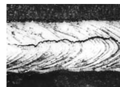
P8 Cold cracks in fillet welds
