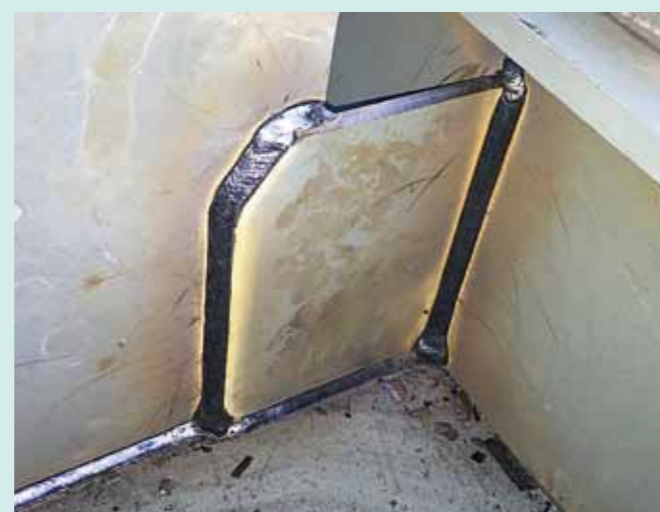
Figure 16: Bead appearance by robotic welding with F DW-100
