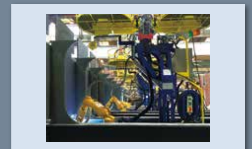
Figure 3: Welding carried out by the ARCMAN™ A30S in the shipbuilding hull assembly
