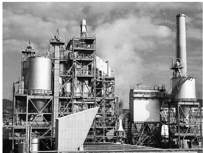
Heat-resistant low alloy steel is a main material for coal firing power plants.
